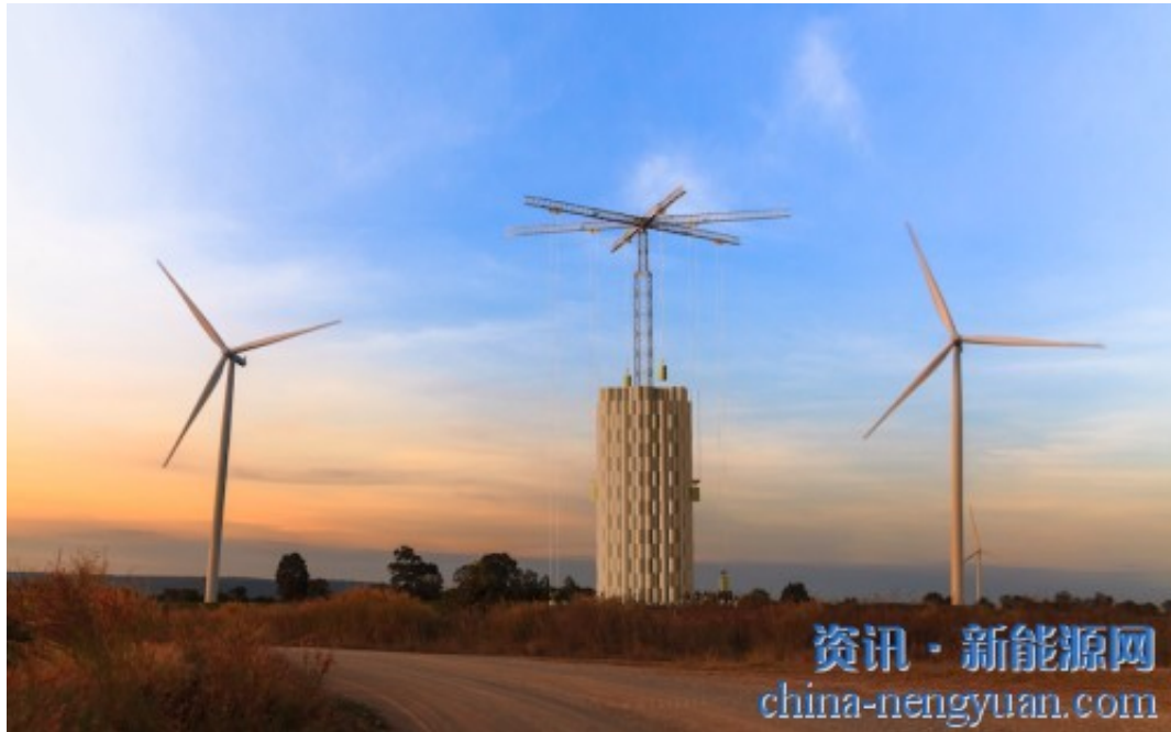
重力储能塔。图片来自：Energy Vault
