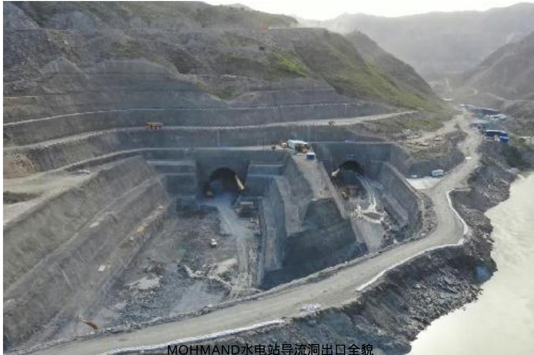
MOHMAND水电站导流洞出口全貌
