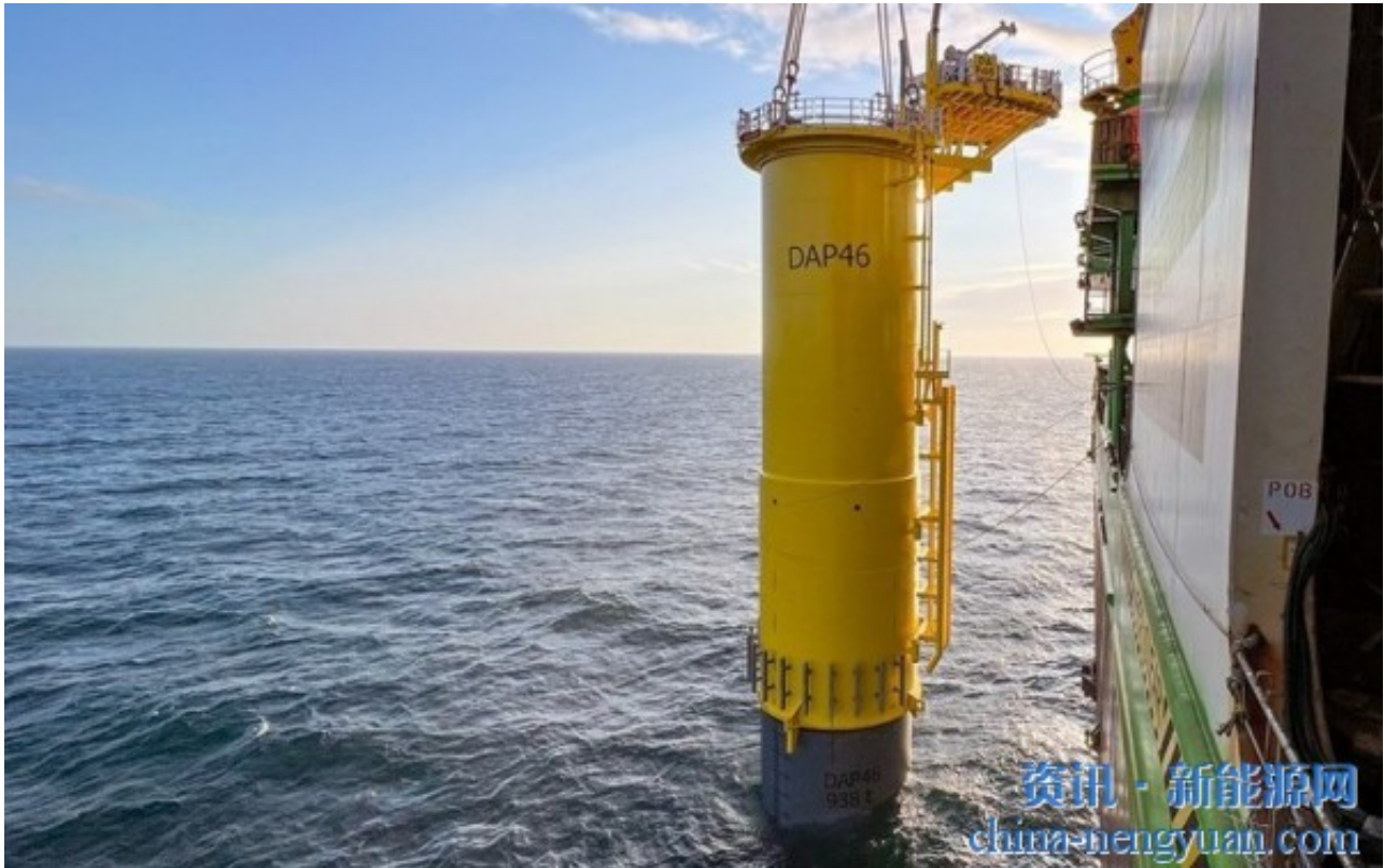
Dogger Bank A风力发电机的桩基。来源：SSE Renewables
