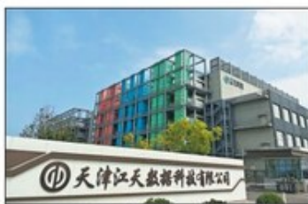
Top: A Tianjin GiantDC Technology Co worker inspects equipment. BY WANGHAO / CHINA DAILY Above: The GiantDC office building in Tianjin. PROVIDED TO CHINA DAILY
